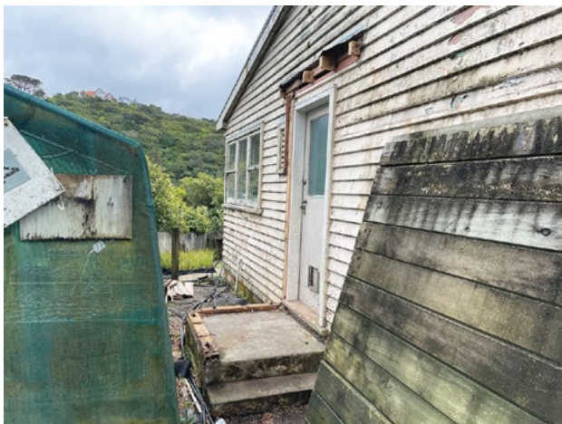
The work gets going. Below: the little porch has been removed prior to the works. Top right shows the state of the existing paintwork and right we can see some of the progress that has been made so far in removing the paint.
