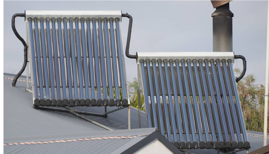
Solar hot water
